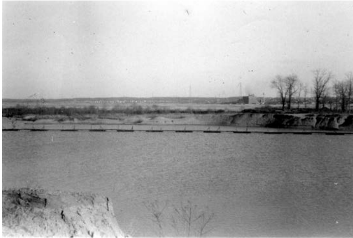
Pic 11. Pipeline carrying slurry of sand and water from the dredge to collection hopper located on Mill Road. (Author's Collection – March 1946)
