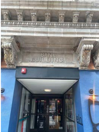
8- Original Bank Building at 406 Main Street (Present day Optique Unique)
